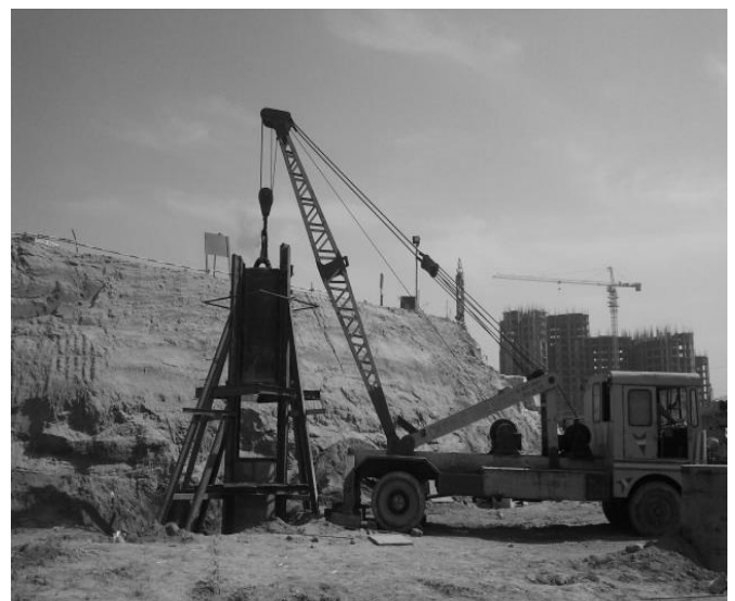
Figure 8. Dynamic Pile Load Test Setup
